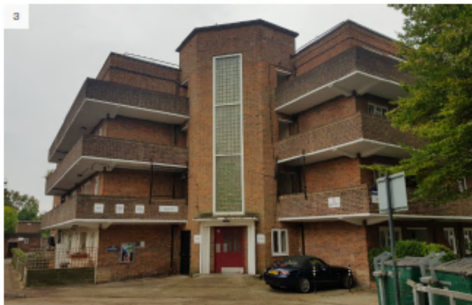
3. View of Entrance Core to existing block 1-20
