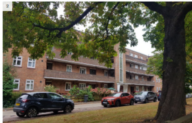
2. View of Existing Blocks to Valentine South facing Perry Vale
