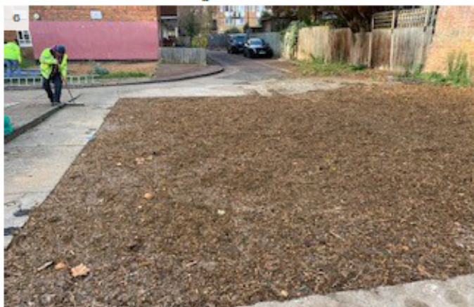
6. View of demolished caretaker block location and access road beyond
